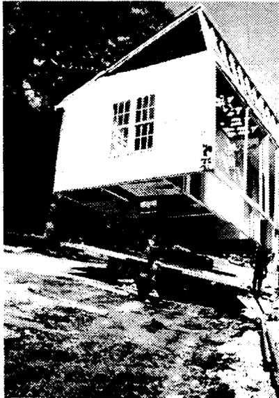
**Figure 2. Modular Box Being Lifted from Removable Floor System.**
