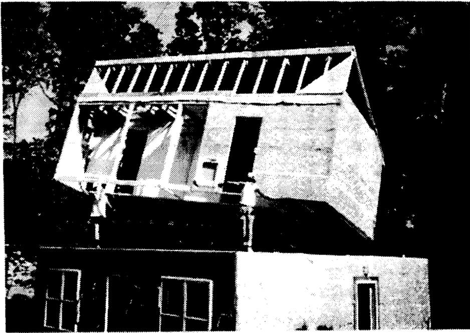
**Figure 7. Floorless Second Floor Box.**
