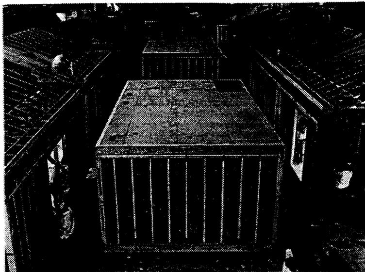
Figure 1. Modular Units Showing Floor and Ceiling on Each Box.
