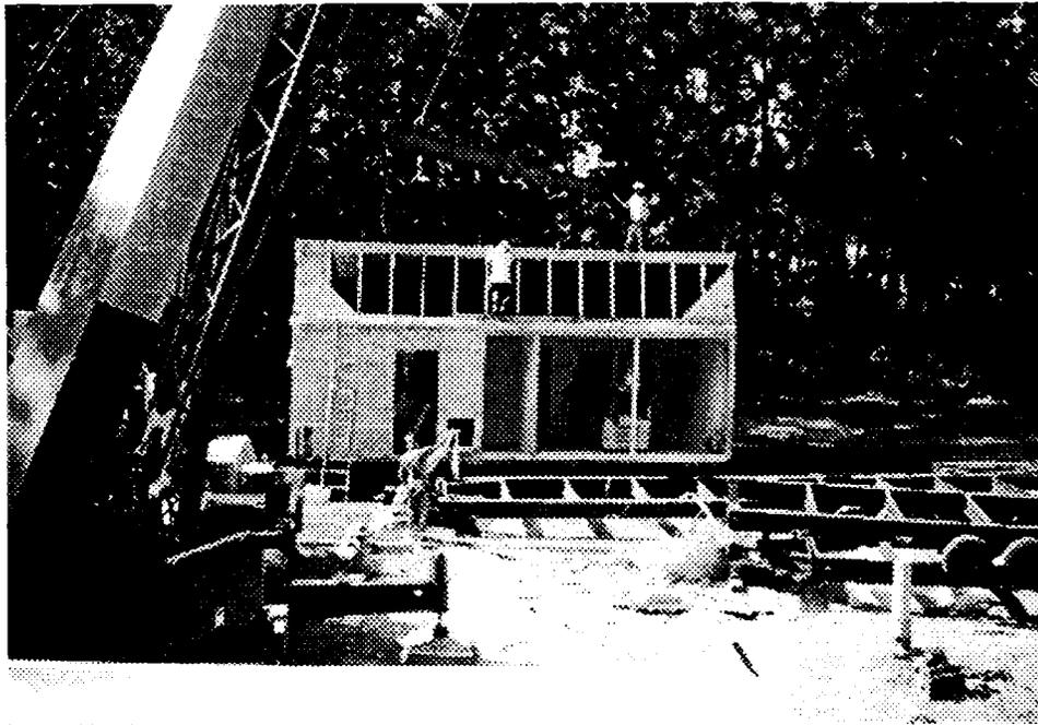
**Figure 6. Lifting of Box**
