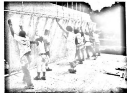
HUD staff help frame a Habitat for Humanity house
