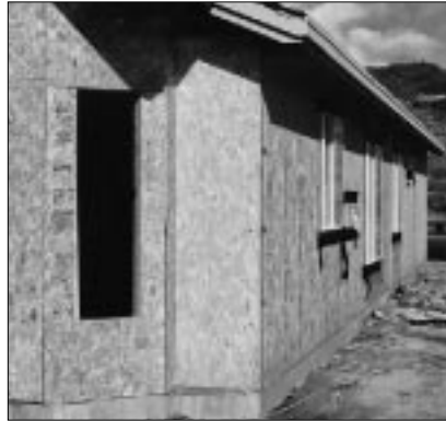
Crown Hills, constructed by a production builder who uses SIPs on a regular basis, appears to be composed of conventional frame houses. SIPs can be pre-cored in order to run plumbing and electrical conduit.
