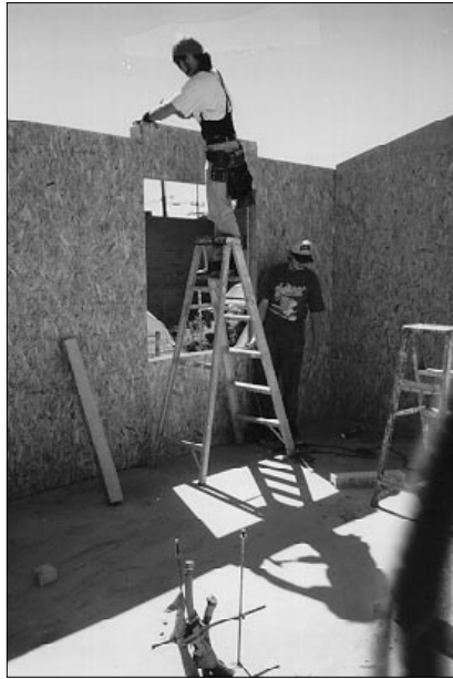
Houses are assembled by at-risk and unemployed local youth, building skills while using SIP construction. Panels can be moved by hand as well as by crane, and are used for walls and roofs.
