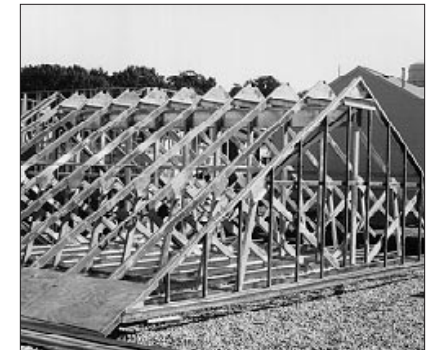
Steel-frame components—such as roof structure and walls—were in some cases preassembled and then positioned by work crews and cranes. Houses were finished with durable, low-cost and low-maintenance materials.
