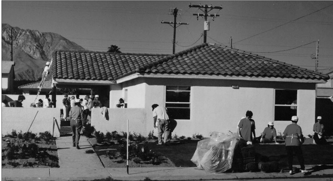
This project uses a steel-framed wall panel system which is infilled with panels of foamed concrete. The light-weight panels can be lifted into place and fastened by unskilled work crews. Steel is also used for concrete foundation forms.
