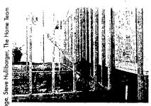
Example of panelized garage built on site. Panelized garage walls set on found dation adjacent to a manufactured home.
