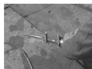
Fig. 3.53: Cutting off misplaced anchor bolt
