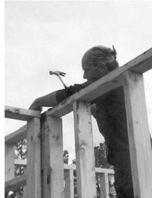
Fig. 3.56: Tying top plates together
