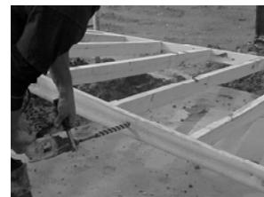
Fig. 3.51: Drilling baseplate for anchor bolt clearance, sill seal gasket in place
