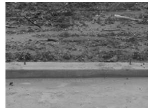
Fig. 3.57: Anchor bolts set too close to slab edge for flush fit between foundation and OSB sheathing
