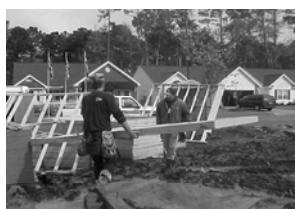
Fig. 3.48: Panels being shuffled at delivery pallet to find needed panel
