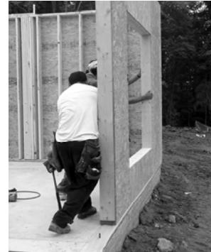
Fig. 3.29: Placing panel over anchor bolts
