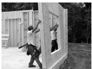
Fig. 3.27: Seating over anchor bolts
