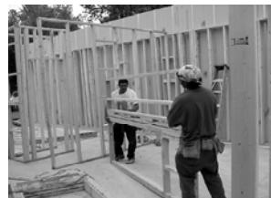
Fig. 3.33: Carrying interior unsheathed wall panel
