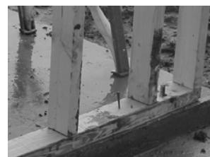
Fig. 3.55: Cut nail temporary anchors
