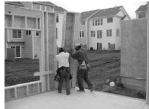
Fig. 3.31: Placing small exterior closure panel
