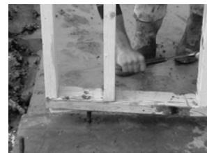
Fig. 3.52: Seating wall panel over anchor bolt
