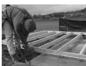
Fig. 3.50: Transferring anchor bolt location to panel
