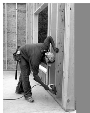
Fig. 3.32: Nailing to adjacent panel
