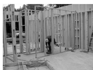
Fig. 3.34: Anchor nailing interior panel to slab
