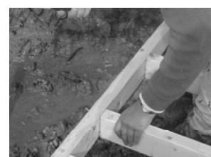
Fig. 3.54: Repositioning stud to avoid interference with anchor bolt
