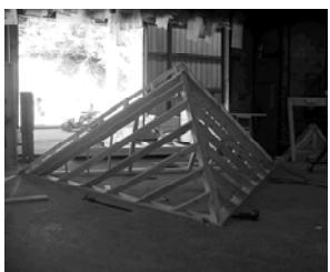
Fig. 3.11: Exterior ready stockpile of dormers
