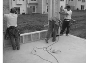
Fig. 3.30: Anchor nailing into position
