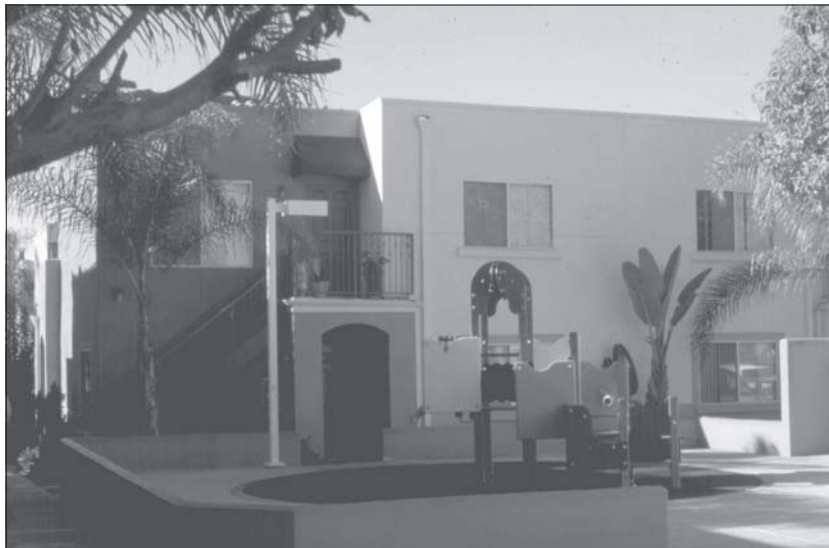
Mercado affordable rental apartments in San Diego, California. The density for this project is 37.3 dwelling units per acre.
