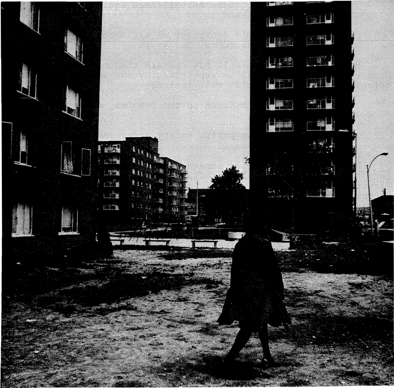
Figure 3.--A view of highrises in Cochran Homes, St. Louis, Missouri
