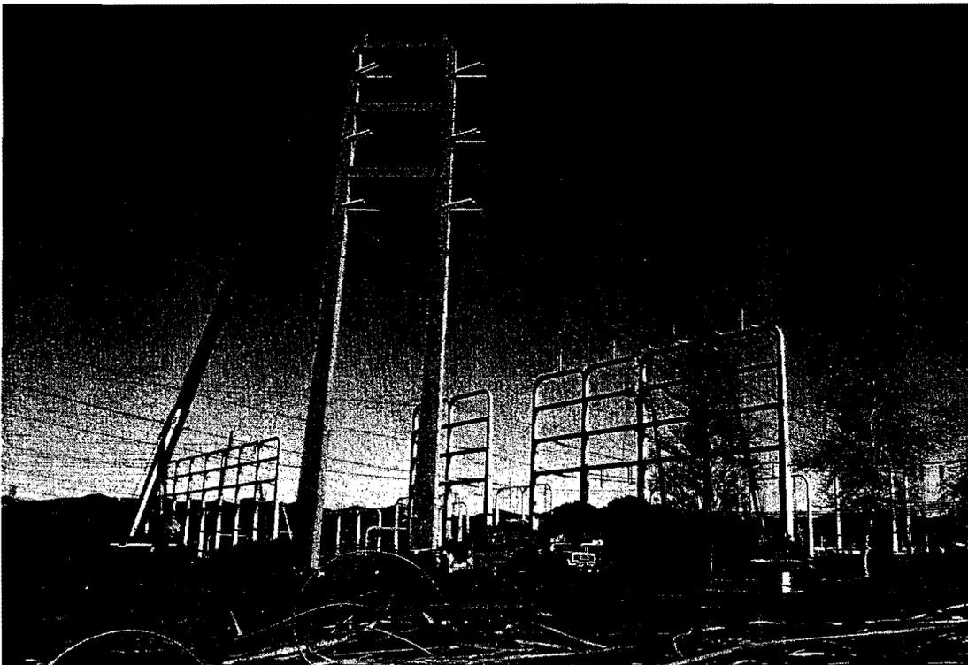
**EXHIBIT 10** Conductor removed from a disabled tower at Pardee Substation, Santa Clarita, CA.
