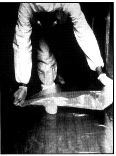
Figure 8.4 Apply a Second Layer of Plastic.
