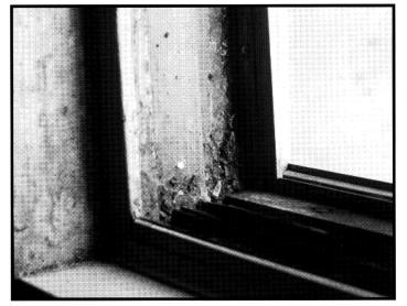
Figure 5.3b Deteriorated Window Troughs Often Contain High Levels of Lead-Contaminated Dust.
