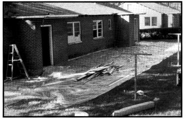
Figure 12.7a Line Walking Surfaces With Plastic.
