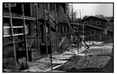
Figure 12.6 Exterior Siding Removal and Replacement.
