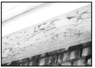
Figure 5.2b Forms of Paint Deterioration: Scaling, Cornflaking, and Peeling.
