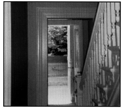
Figure 18.3 Historic Property Where the Interior Woodwork and Staircase Were Wet Sanded and Recoated With Three Layers of Encapsulant To Preserve the Carved Profiles.
