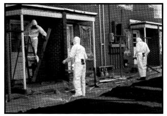
Figure 12.3b Remove and Replace Trim (exterior).
