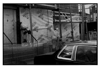
Figure 12.10a Use of Tyvek on Building Exteriors Prior to Enclosure.
