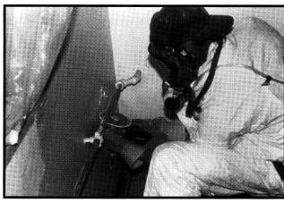
Figure 12.12b Open-Faced Power Sanding or Grinding Is Prohibited.
