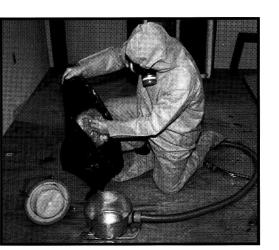
Figure 11.16d Tape Vacuum Bag Closed and Put Inside Plastic Trash Bag.
