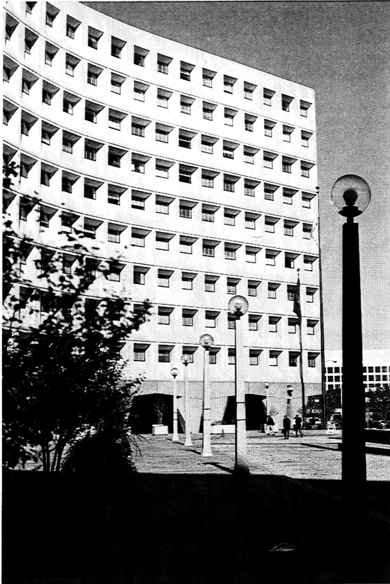
Illustration No. 4-4 Subject: Housing and Urban Development Building, Seventh Street (East) Elevation Date: November 1994 Description: View looking north across plaza (see Illus. No. 3-47 for original view). Changes to the plaza include the removal of concrete stanchions and addition of plants set in concrete landscaping planters, removal of original light fixtures and replacement with clear glass globes set on original concrete standards, new spotlights mounted on the tree beams on the building, a concrete paved driveway area with a granite curb instead of the original bluestone which covered the entire plaza, and two new 80' flagpoles at the north and south ends. Photographer: Reed A. Black, AIA Source: Oehrlein & Associates Architects
