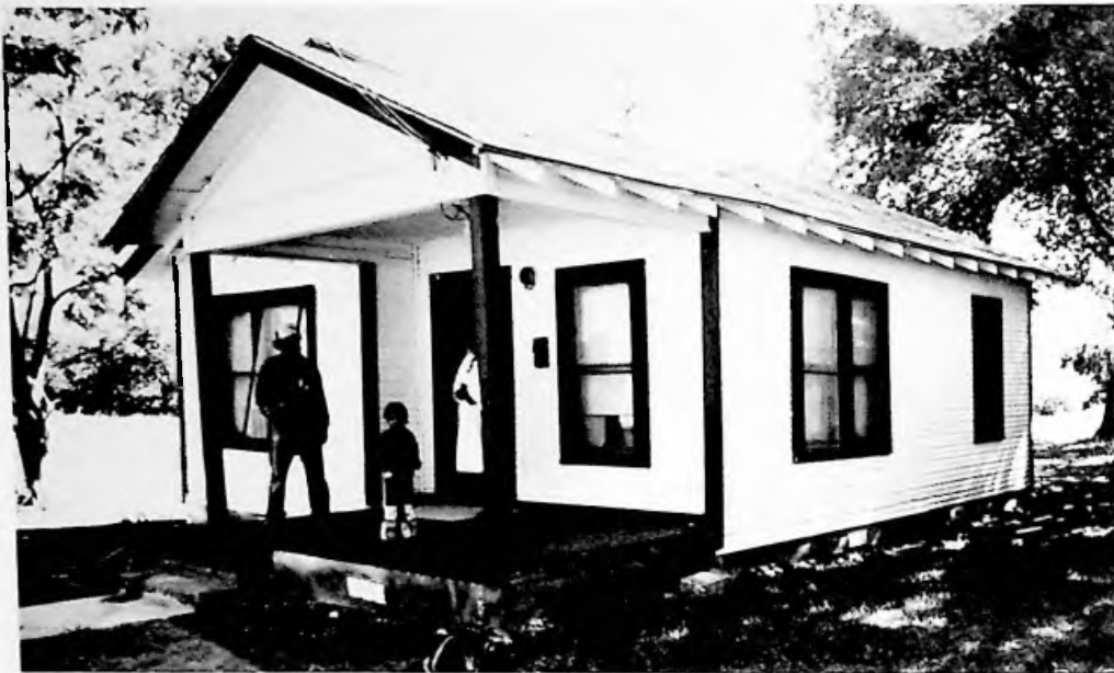
Before Common Ground renovated it, this house looked ready for the bulldozers. Now it once more provides a decent, safe, and sturdy home for a low-income Dallas family
