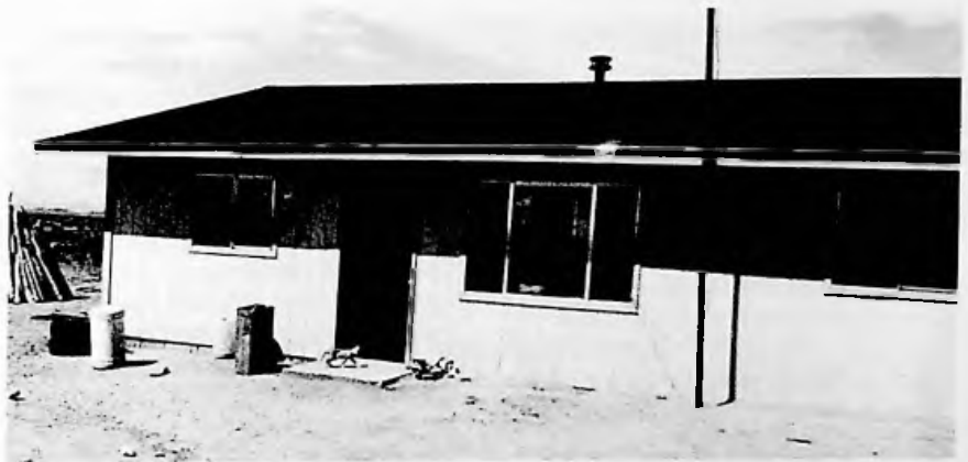
The homes built by UNDC have no frills--just two or three bedrooms, a living room, kitchen, and bathroom built on a 4-inch slab--but they provide warm, sturdy shelter.
