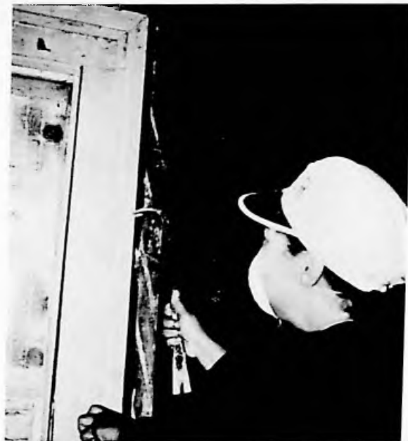
Grace Muhammed removes the old lath and plaster to prepare for the installation of new fire-proofed, insulated walls.
