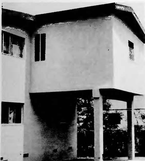
This eight-unit rehabilitation project involved a second floor bedroom addition. Even major renovations like this one were accomplished without displacing tenants. Tenants participated both in renovation planning and execution.
