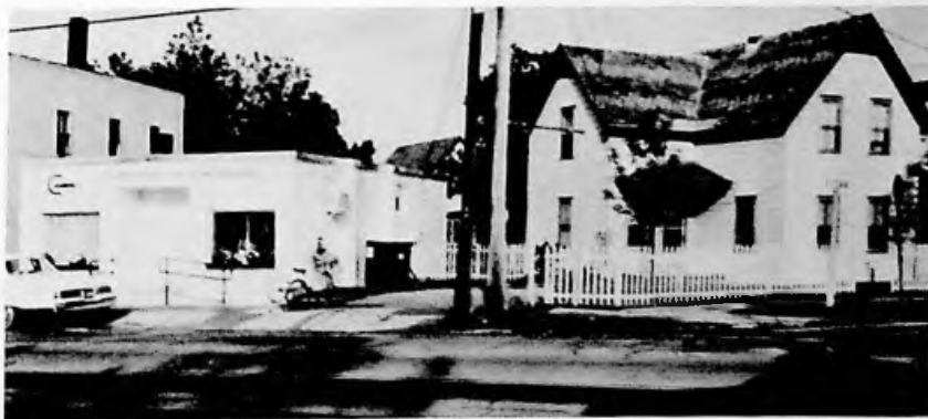
The newly renovated Community Health Center serves a large population in an old section of Burlington. The Land Trust bought the property and obtained loans from the Institute for Community Economics and the Sisters of Mercy to finance the rehabilitation. The Burlington Youth Employment Program did the work. The house to the right was also renovated through a partnership between the Land Trust and BYEP.
