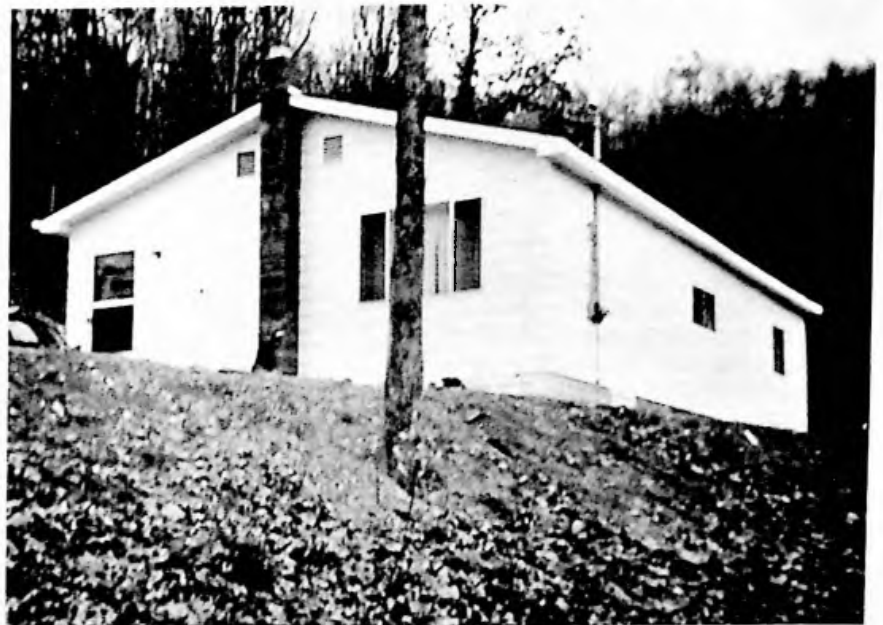
It's hard to believe these are photos of the same house. Reid Hatfield's Clay County home lacked just about everything. Kentucky Mountain Housing totally rebuilt it, insulated it, added a living room, and drilled a well. Use of trainee labor and low-cost construction techniques kept the total rehabilitation loan down to only $5,000.
