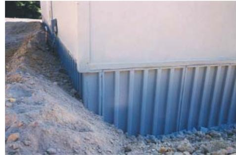
Figure 4.14 The coated panels can safely be backfilled.
