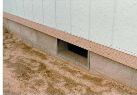
**Figure 2.10** Foundation wall detail showing an air vent.
