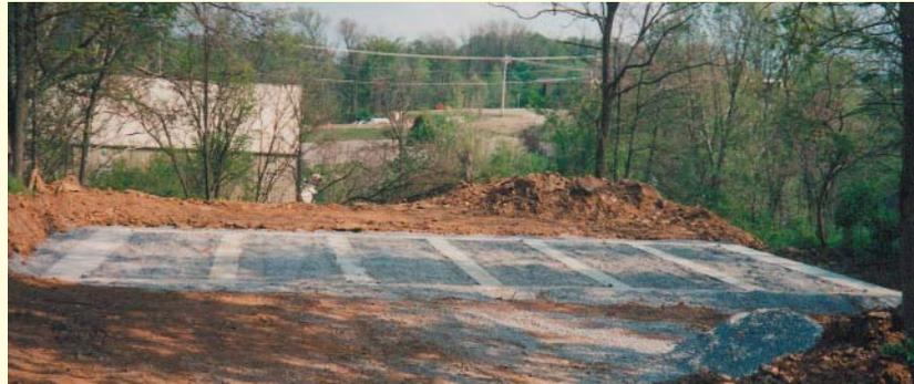
**Figure 3.25** Open cells filled with crushed rock.
