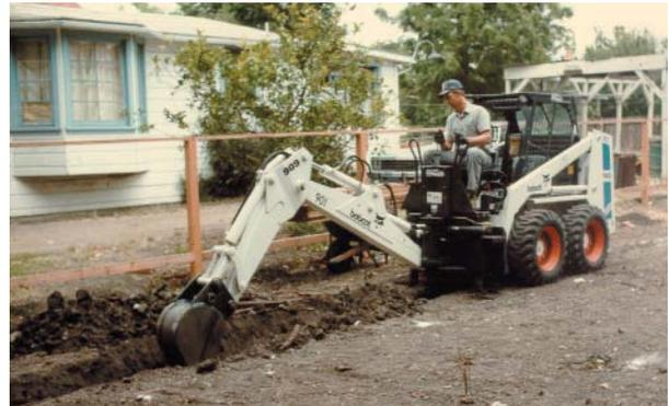
**Figure 3.12** Excavating for perimeter footings with a backhoe.
