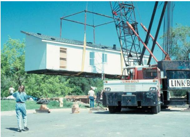
**Figure 3.17** Installing a home with a crane.
