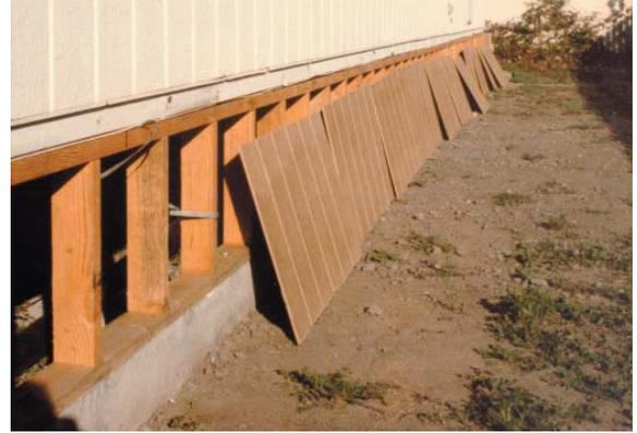
**Figure 3.15** Ponywall construction method.
