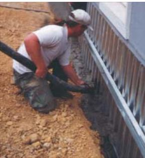
**Figure 4.12** Concrete added to the trench.
