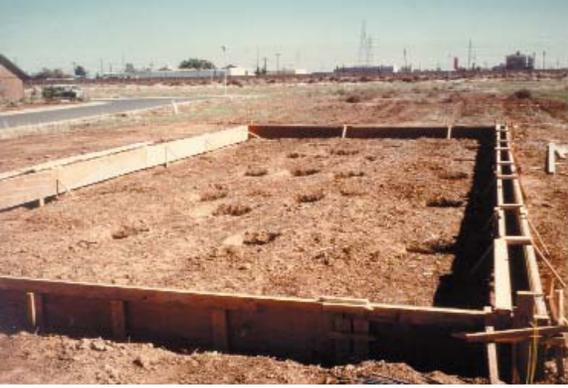
**Figure 3.14** Forms ready for concrete pour.
