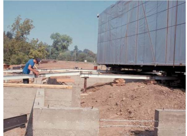
**Figure 3.18** Installing a home with a roller system.
