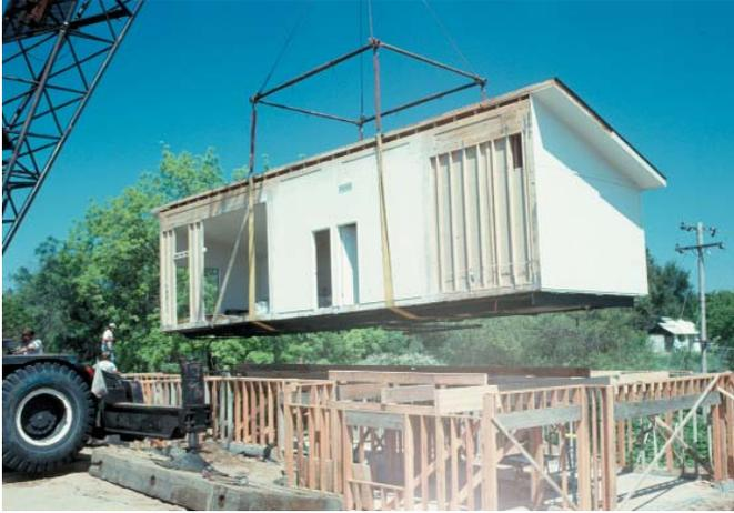
**Figure 3.66** Above-ground basement with garage.
