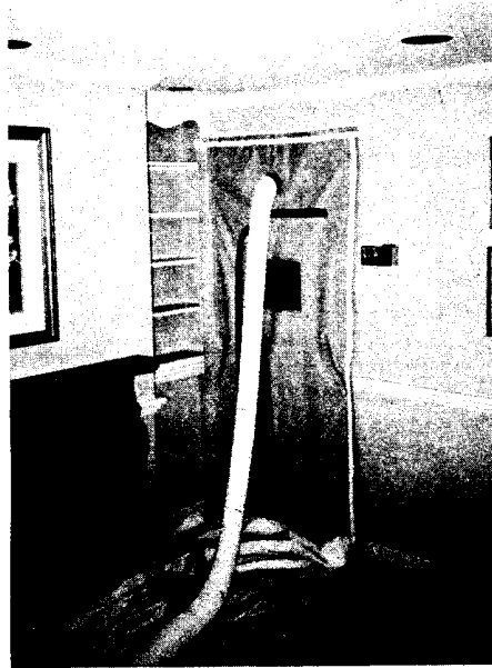
Photo 4. Construction Dust Control
