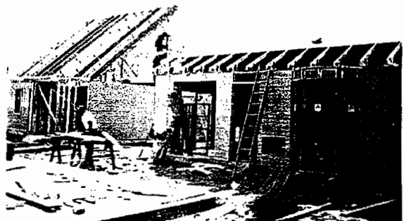
Units under Construction
