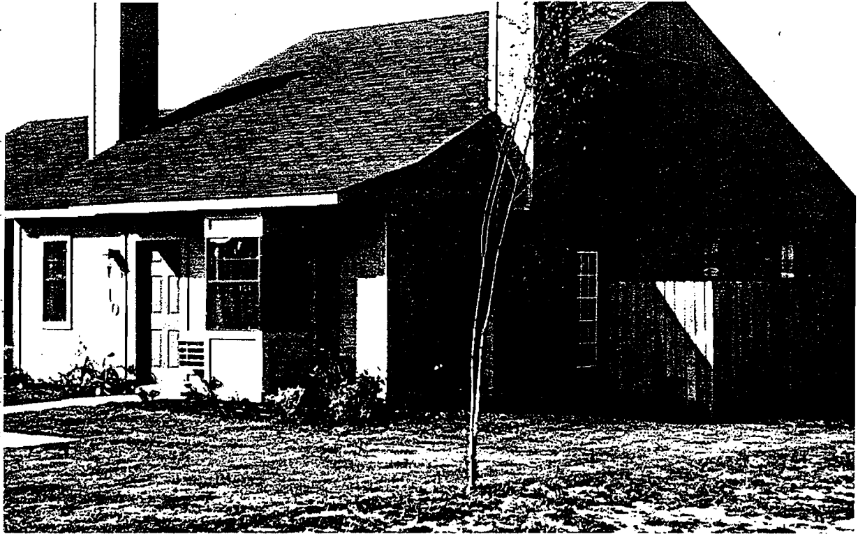
Exterior of 3-bedroom unit.
