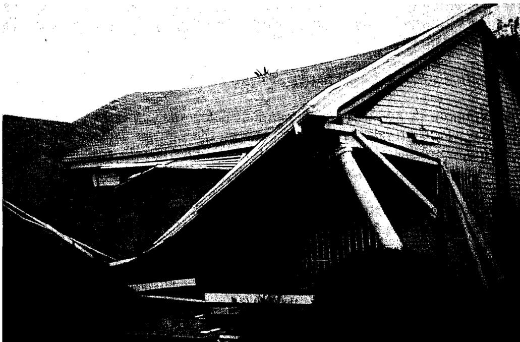
**EXHIBIT 8** The result of cripple-wall failure in a wood-frame house.
