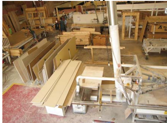
Figure 23 Gypsum board cutting station and new storage rack for cut gypsum board
