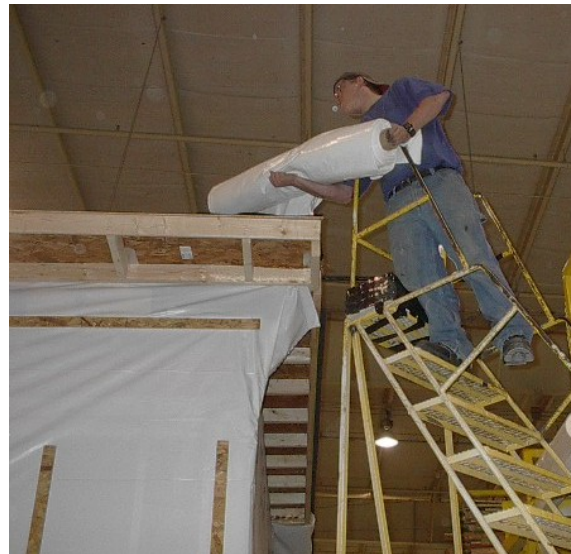
Figure 54 Lifting a roll onto the roof
