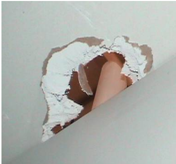
Figure 42 Vent pipe punch out
