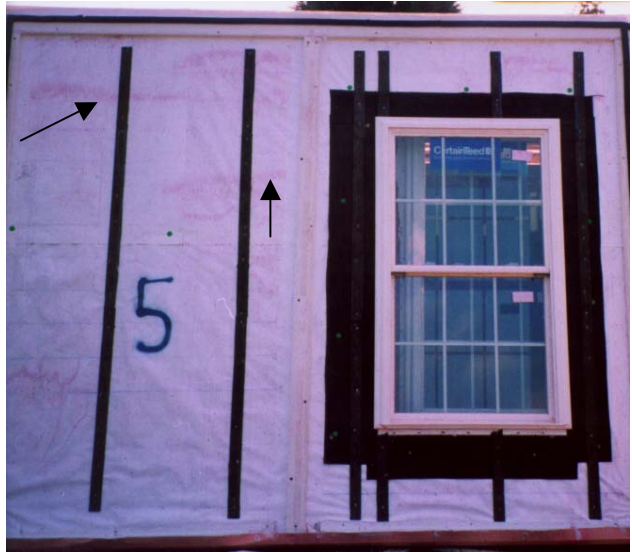
Figure 14 Fiber Cement with Drainage Plane
