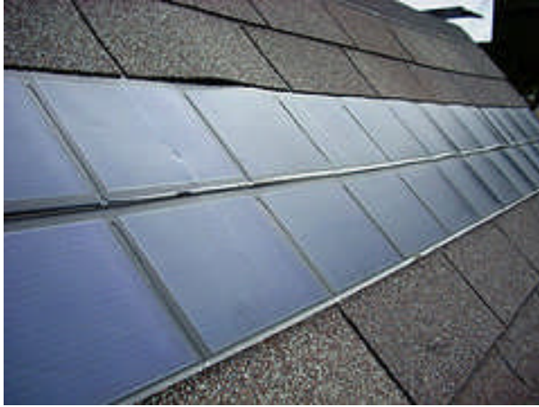
Solar Shingles on residential roof, one of many solar features. Source: Flickr
