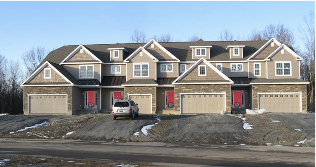
Guarded blower door testing, with a blower door on the doorway of each townhome, is expensive and impractical, because construction on the entire building must be temporarily halted. Photo credit: Newport Partners.
