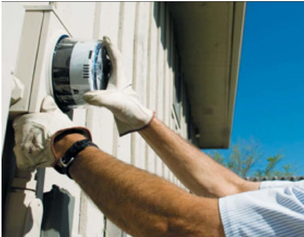
Installation of Smart Meters
