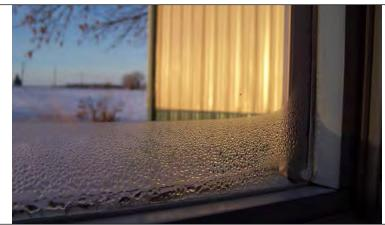
**Good intention:** Weatherized house (added insulation and airtightness). **Unintended consequence:** Amount of indoor humidity and window condensation became elevated. **Solution:** Control interior moisture sources; add source point and whole-building ventilation.
