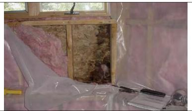
**Good intention:** Framed wall with good insulation, air barrier, and vapor retarder. **Unintended consequence:** Water leaked into a window cavity that had limited drying potential. **Solution:** Provide proper exterior water management to limit water infiltration.
