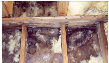
**Good intention:** Heavily insulated wall cavities and rim (band) joists. **Unintended consequence:** Air-transported moisture (because of elevated interior humidity and indoor pressures) condensed on the cooler sheathing. **Solution:** Install a continuous air barrier to prevent exfiltration of moisture air during winter.
