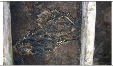
**Good intention:** Constructed 2-x-6 frame walls with good insulation, air barrier, and vapor retarder. **Unintended consequence:** Improper stucco cladding added moisture to a cavity that had low drying potential because of reduced heat and airflow.
