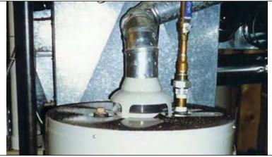
**Good intention:** Ensured the house was well insulated and air sealed and added exhaust devices. **Unintended consequence:** Negative pressure in the combustion zone caused backdrafting of combustion byproducts into the house.
