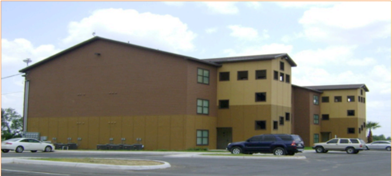
Figure 12. Energy Lodge, Carrizo Springs, Texas
