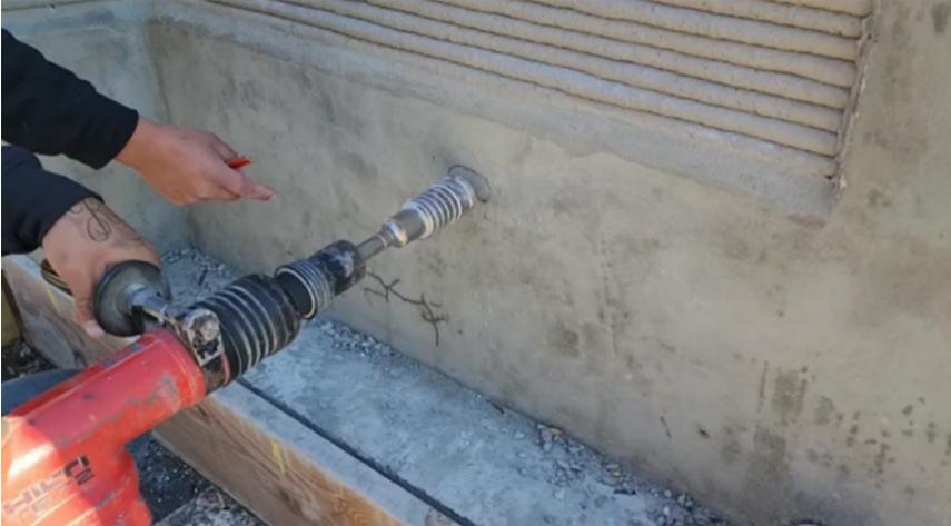
Close-Up of Drilling for Plumbing. Photo credit: Home Innovation Research Labs (2022).
