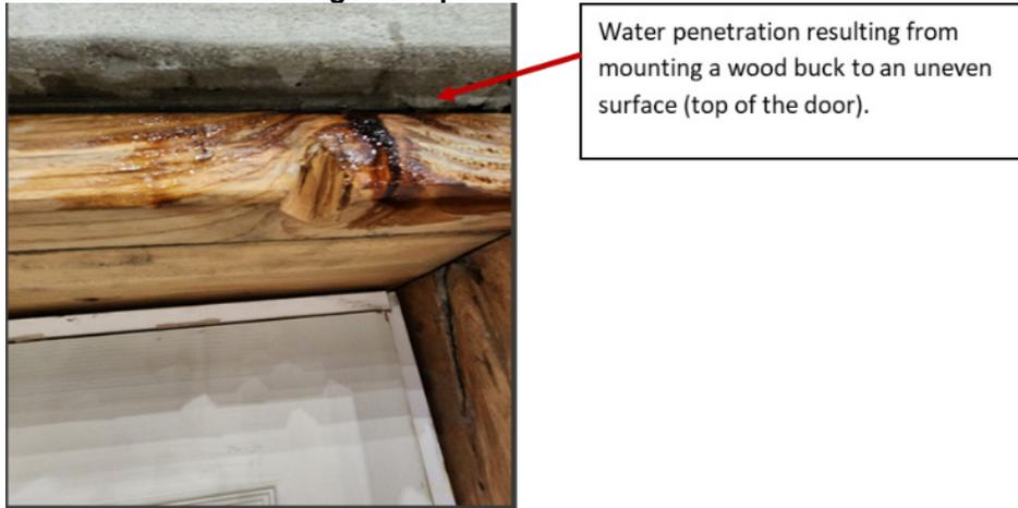
Close-Up of Door Inspection Leak. Photo credit: Home Innovation Research Labs (2022).
