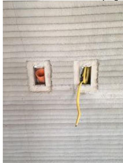
3D Printed Wall with Close Up of Utilities.
