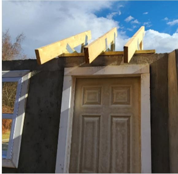
Roof Structure Mounting Detail.
