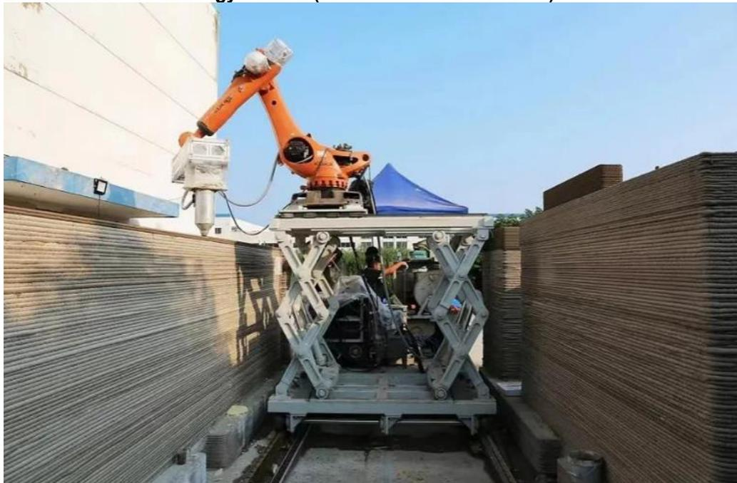
RIC 2 Robot Constructing Wall. Photo credit: RIC Technology (2022).
