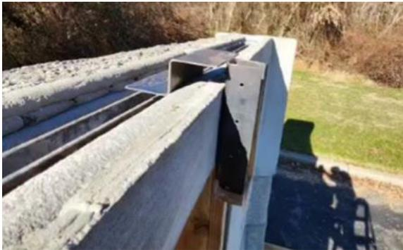
Custom Installation of Joist Hanger. Photo credit: Home Innovation Research Labs (2022).
