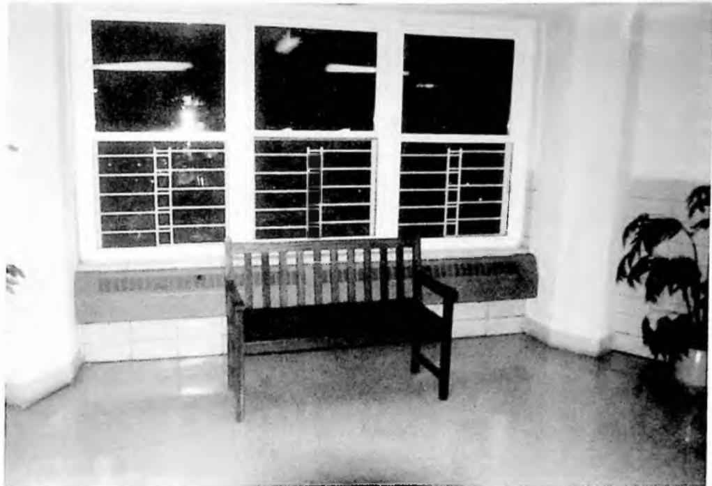
The interior hallway is well lit. Existing glazed block was cleaned for reuse because of its durability and easy maintainability. Lead-based paint on hallway walls was encapsulated with a product which leaves a stucco-like finish on the walls.
