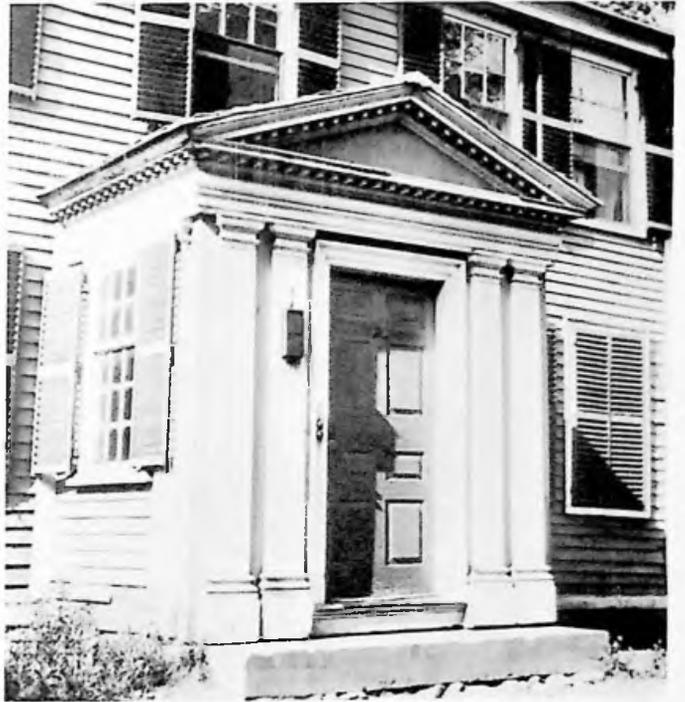
*John Bemis House, Massachusetts (ca. 1740). This is an unusually large and elaborate vestibule complete with shuttered windows. Vestibules are generally unheated spaces not requiring this heavy construction.*
