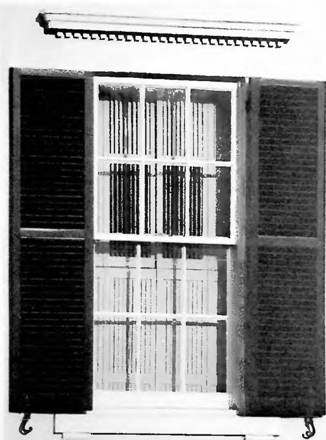
*House, District of Columbia (late 19th century). These shutters have fixed louvers, designed more for filtering the sun than for reducing heat loss. Notice the hardware for holding the shutters open so that they do not swing freely. The interior shutters have adjustable vertical slats.*
