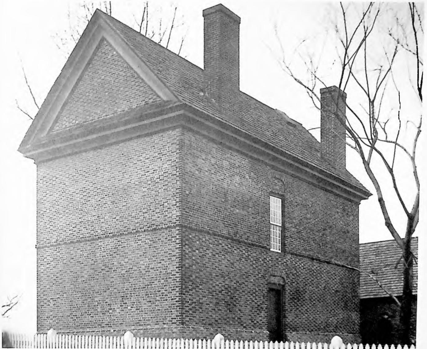
*Bel Air (Singlev House), Pennsylvania (ca. 1725). The north elevation of this house has no windows except for one which lights the stair landing. There are two interior chimneys in the north wall with fireplaces flanked by closets in each room. The coldest wall in the house is thus isolated from the inhabitants. The closets also serve as warm air convection flues to provide additional heat.*
