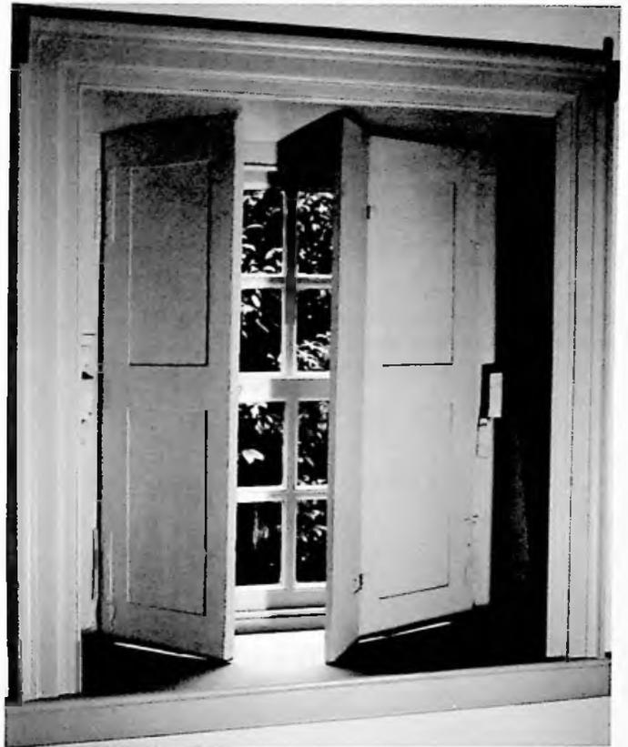
*Stratford Hall, Virginia (ca. 1730). Interior shutters, as opposed to exterior shutters, are designed to be invisible when open. Unfortunately, they are frequently stuck in the open position by accumulated layers of paint. This same window is illustrated with the shutters open in the section on splayed window reveals.*
