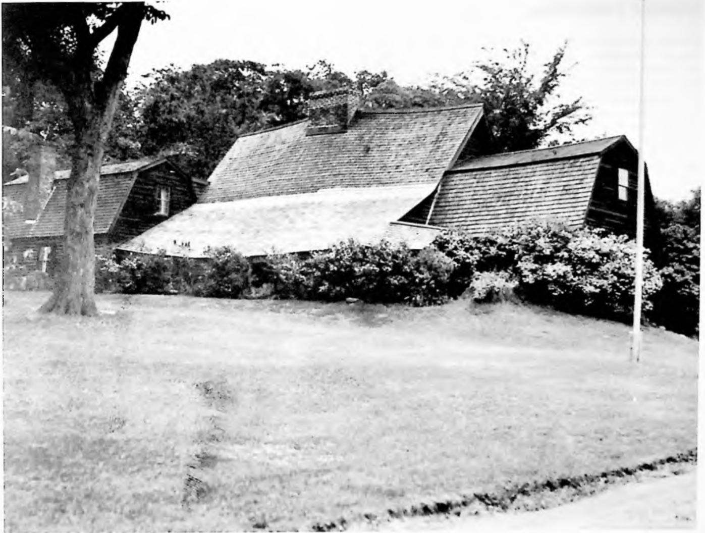
*Fairbanks House, Massachusetts (1636). The house is nestled against the southeast slope of a hill with a berm and dense shrubbery protecting the north and west walls from the New England winters. Notice how little of the house other than the roof is visible in this view from the northwest.*
