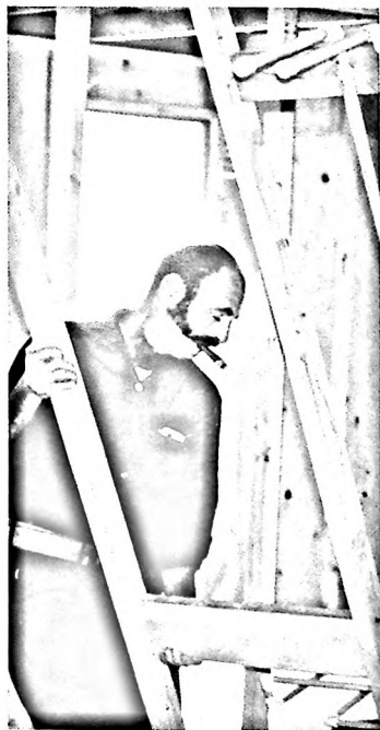
Workmen at the OVE research house in Maryland install the prefabricated plumbing wall containing plastic pipe. The NAHB Research Foundation designed the cost-saving techniques used in the house.
