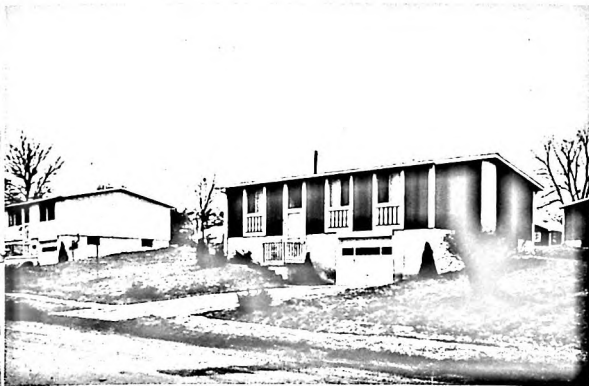
HOME BUILDING CORPORATION uses factory-built modular units made of wood, which are applicable to single-family detached dwelling units, single-family attached dwelling units, and multifamily low-rise dwelling units.
