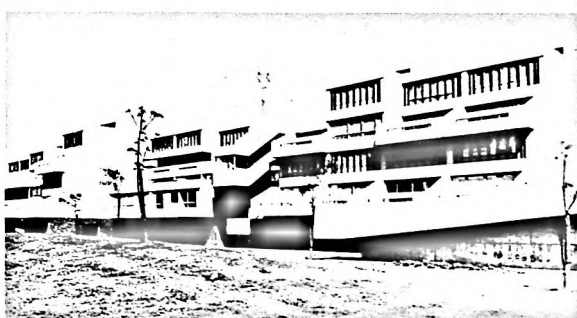
HENRY C. BECK COMPANY is introducing to the American market the Balency precast concrete system which uses factory-produced concrete floor and wall panels. The system can be assembled on site into all types of housing from single-family detached to townhouse, deckhouse, or high-rise dwellings.
