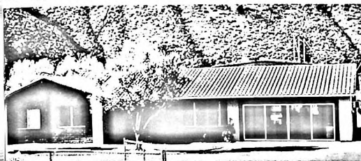
SHELLEY SYSTEM uses a factory-produced concrete modular system, in a multifamily low-rise building to demonstrate a system applicable to multifamily low-rise dwellings, multifamily high-rise dwellings, and adaptable to single-family attached dwellings.
