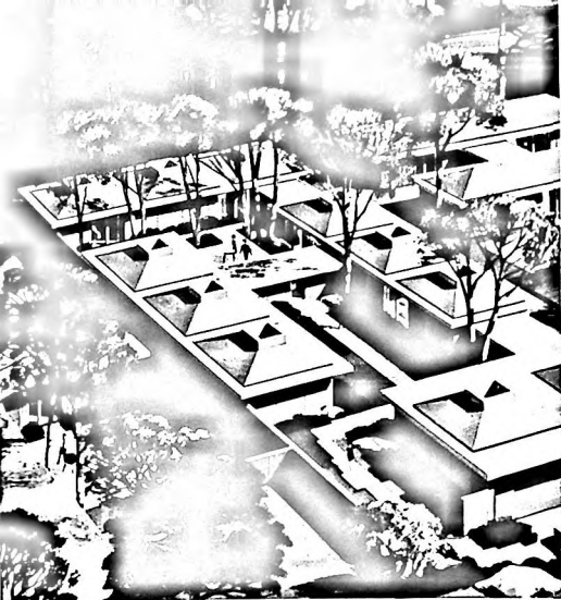
REPUBLIC STEEL CORPORATION'S single-family detached dwelling can be assembled on site from factory-fabricated panels and components. Using steel as the principal structural material, these components are formed into one or more modules with a self-contained mechanical system.
