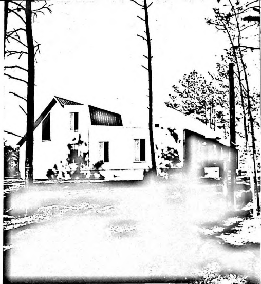
HERCULES INCORPORATED uses wood-framed, single-family units that are assembled from factory-made wood modules and accessory parts. Single-family attached and multifamily low-rise dwellings are also possible with this system.
