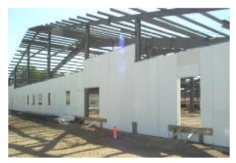
Aluminum and steel-rib panels in construction
