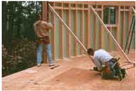
Wood-based open-wall system is the closest technology to conventional stick framing
