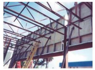
Roff structure frames into concrete panels
