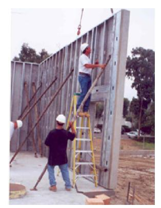
Concrete panels have open-wall of steel studs
