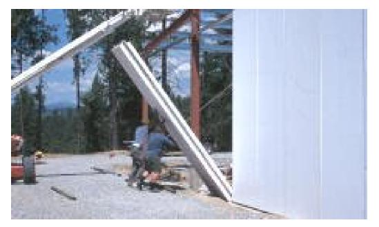
Steel and foam panels are lighter and easier to assemble
