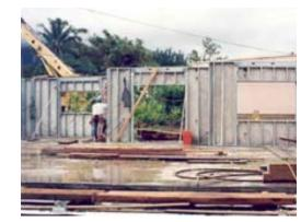
Open-wall system allows access for utilities
