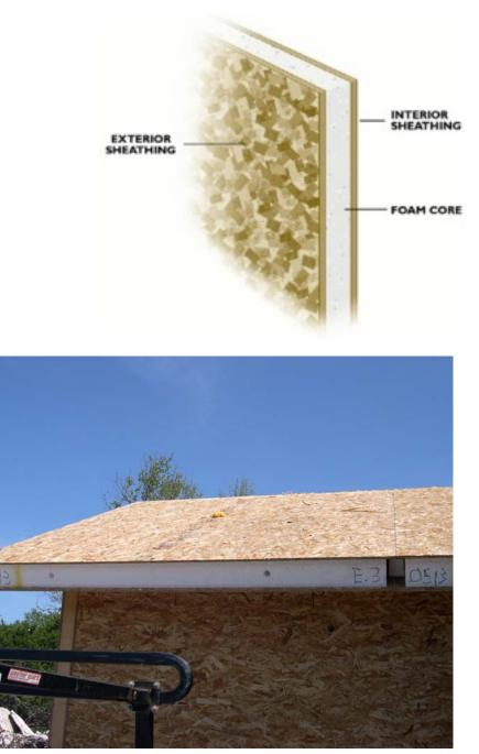
Structural insulated panels are used for roofs as well as walls, with pre-cut channels
