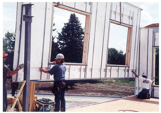
Panels of EPS foam interspersed with steel stud channels
