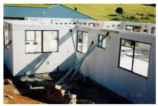
Panels are stabilized by struts during erection process
