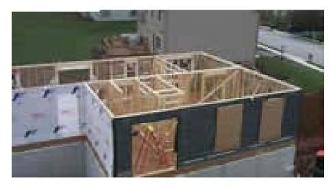
Exterior open wall panels with stick-built interior partitions
