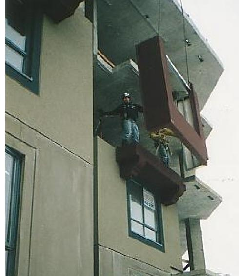
Glass fiber reinforcing provides exception strength in single-unit wall sections
