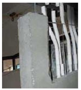
Pipe connections in preformed gypsum panel
