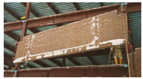
Panel exterior is finished with brick-and-mortar
