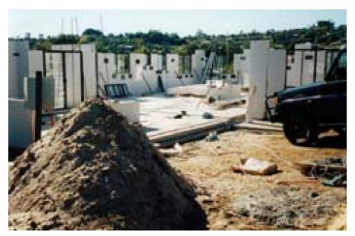
Erection on-site of AAC concrete panels
