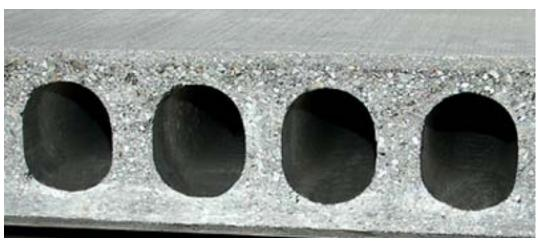
Concrete panel core is hollow for utility chases and to lighten the members
