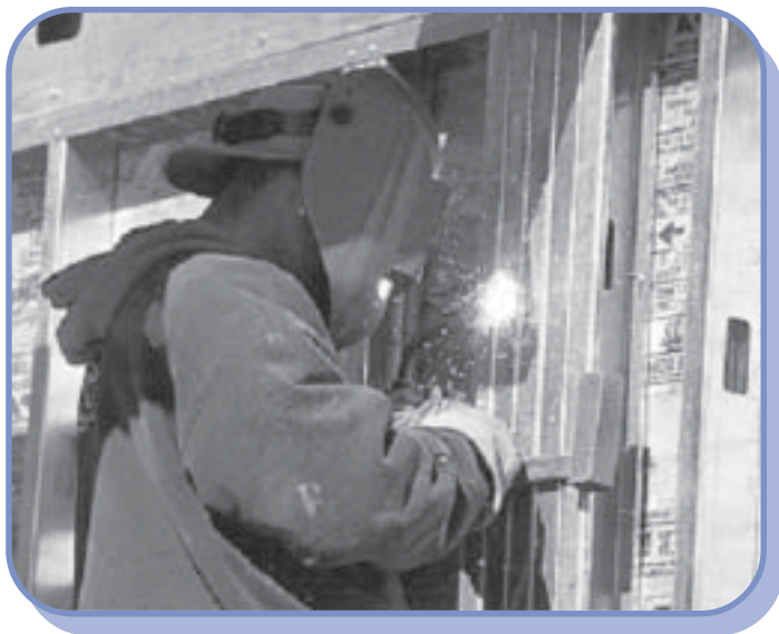
Figure 4.12–Welding of Cold-Formed Steel Framing
