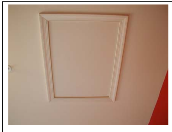
Figure 16 Finished Hatch in Place
