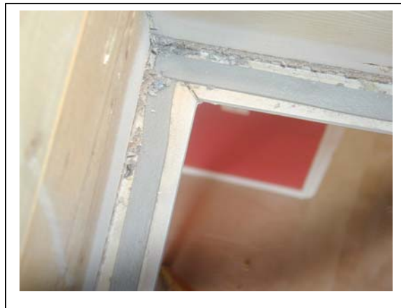
Figure 15 Gasket in Place
