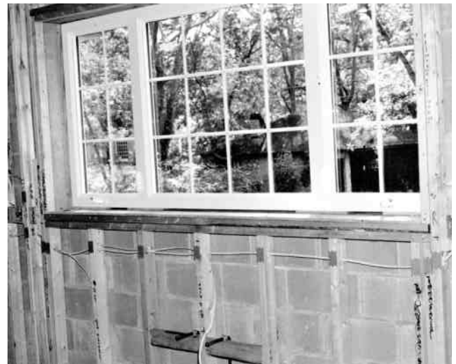
Figure 6-6: Plumbing Rough-In on Exterior CMU Wall
