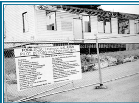
Pilot deconstruction project at Fort Ord, north of Monterey, CA. (Reprinted from Biocycle, November 1998)
