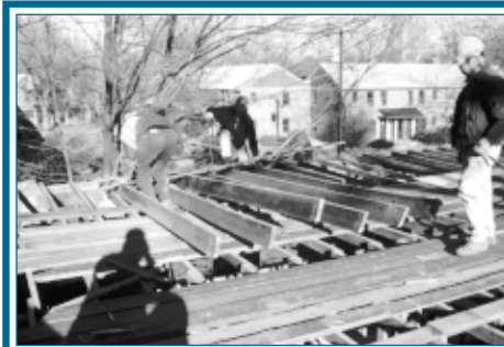
Floor system disassembly
