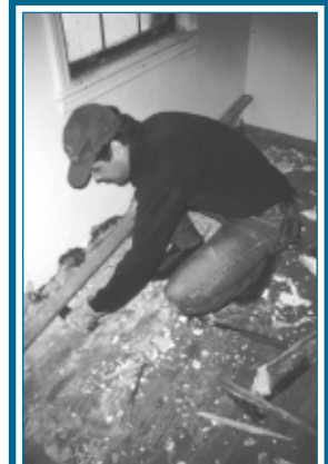
Hardwood flooring removal
