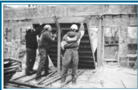
Stair removal – Riverdale Village.
