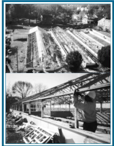
Greenhouse frame disassembly – Walter Reed Army Hospital
