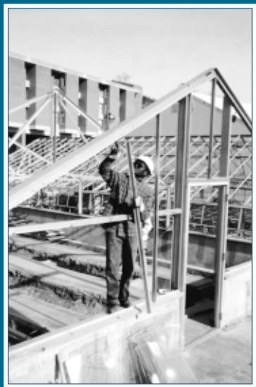
Greenhouse frame assembly— Walter Reed Army Hospital.
