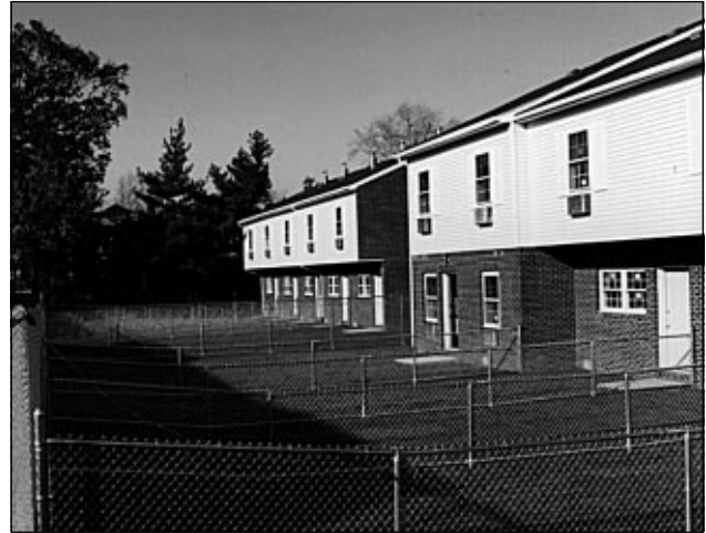
Figure IV-11: The fencing-off of the rear yards in the Yonkers scattered-site housing. Individual yard fences are 3 feet high. The 6-foot fences defining the collective rear yard area can be seen in the foreground and at rear.
