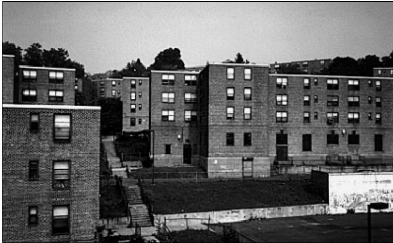
Figure IV-6: Existing public housing in Yonkers: Mulford Gardens.
