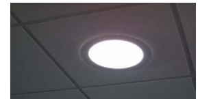
Figure 21: Solar Tube Lighting
