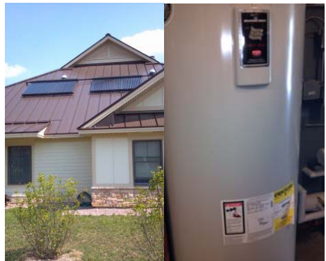
Figure 9: Solar DHW for a Phase 2 building (left) and electric DHW tank (right).
