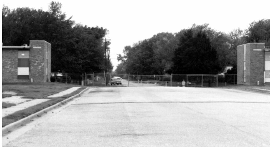
Photo 2.2 Worsening crime led to the erection of fencing limiting access to the property. (Carole Walker)
