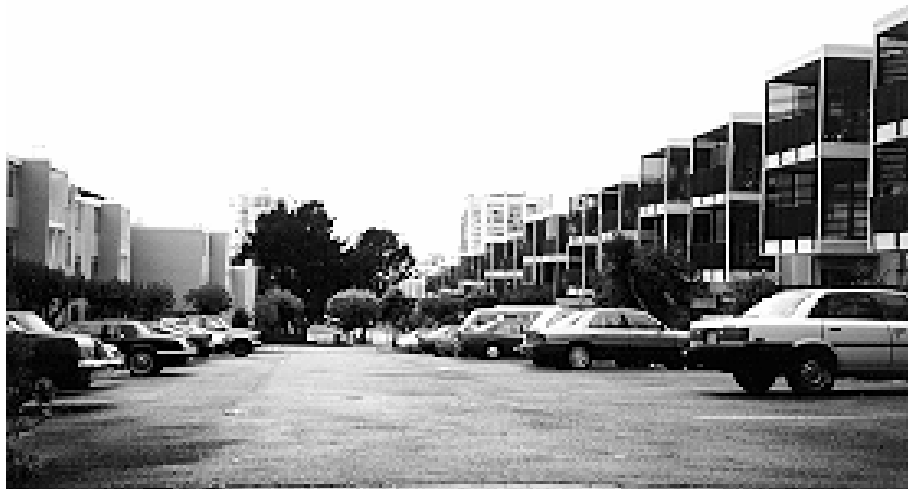
Photo 4.4 Low-rise multifamily development at Old Saint Francis Square, Western Addition. (Joanna Davis)
