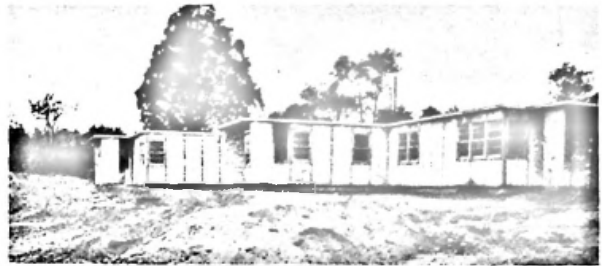
Some of the experimental "rammed earth" houses put up at Alexandria (Virginia) as described above by Mr. Saarinen. (An FPRA photograph.)
