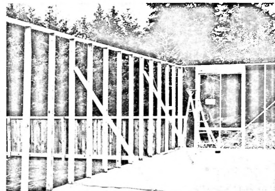
Exterior wall framing
