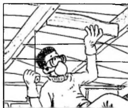
LACING WIRES ON NAILS SET INTO JOISTS
