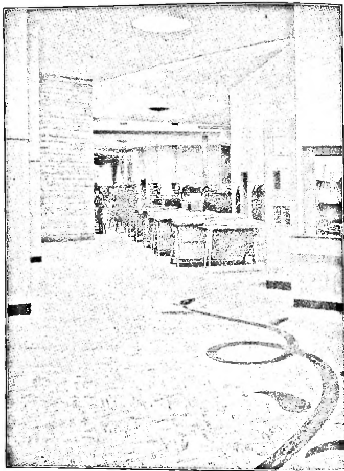
FIG. 31. INLAID RUBBER TILE WITH INSERTS
