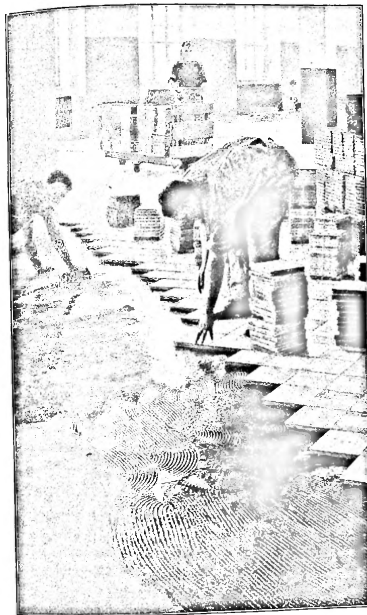
FIG. 35. LAYING UNIT WOOD-BLOCK FLOORING
