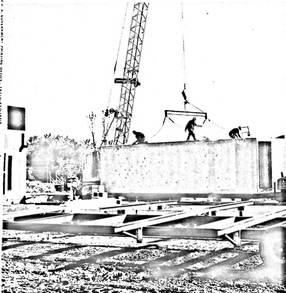
A crane lifts a module containing half a two-bedroom unit into place at Wright Park Manor housing project in Rome, N.Y. This first 200-unit phase of Section 236 subsidized housing is insured by the New York State Urban Development Corporation rather than by HUD-FHA. The NYSUDC has an extensive Housing Technology Program already in operation.
