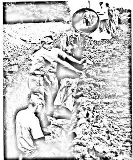
Workmen encased all of the ductile-iron pipe, ranging in size from 16 to 36-inches, in 8-mil polyethylene wrap for additional protection from corrosion.
