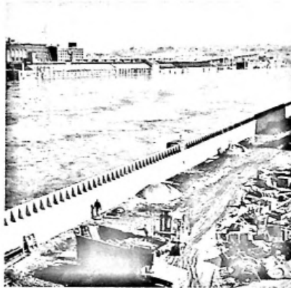
RIGHT —To be eligible for flood insurance under the Federal Flood Insurance Program, a city must agree to take appropriate land use and management actions. Such building codes and zoning regulations would cover protective works such as walls to avoid water damage in the future.
