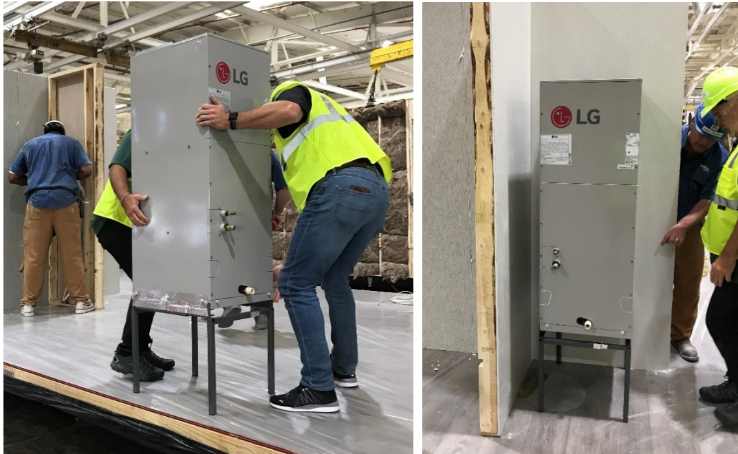
Exhibit 30. LG Electronics Air Handler in Interior Mechanical Closet
