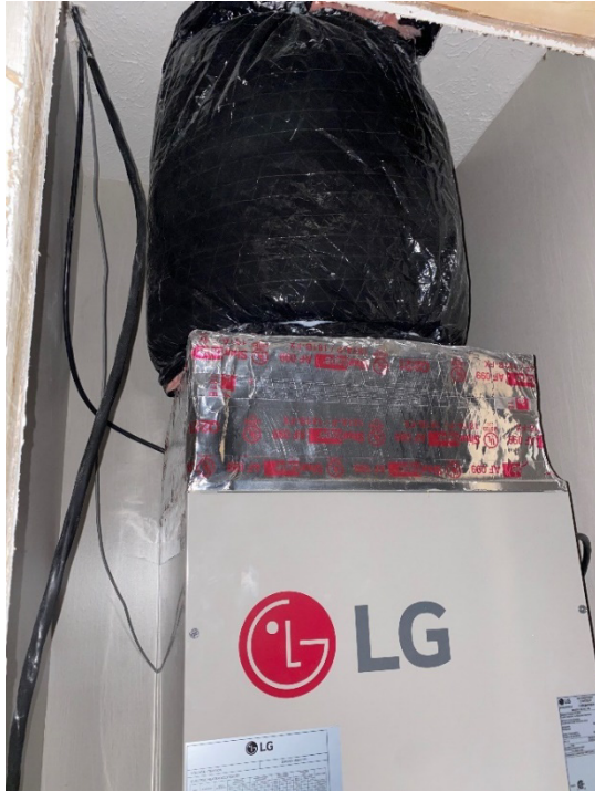
Exhibit 33. Supply Air Ductwork Connection to LG Electronics Air Handler
