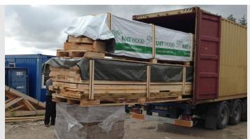
**Precut homes** are a type of factory-built home in which building materials are cut in a factory according to design specifications, transported to the site, and assembled there. Precut homes include kit homes, log homes, and dome homes.
