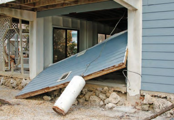
Breakaway wall with no damage to structure.
