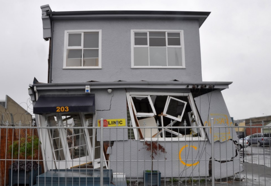
Failure due to lack of drag struts.
