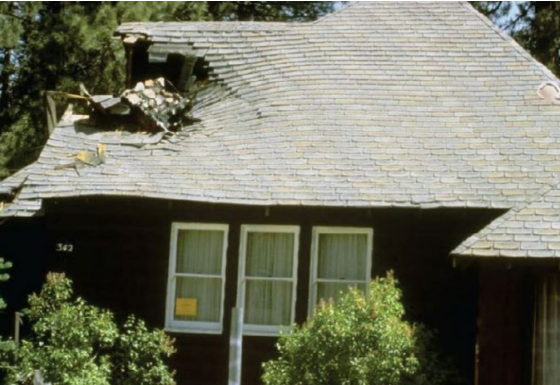
Chimney failure.
