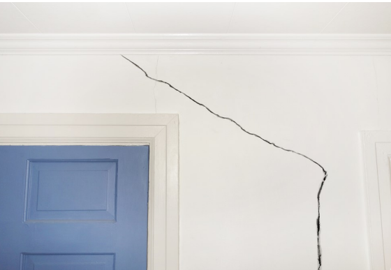
Drywall crack.
