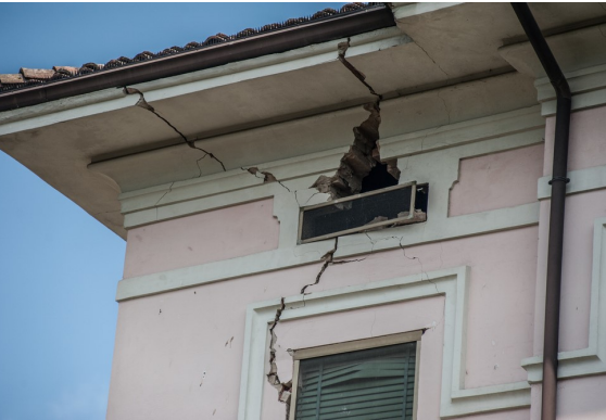
Wall cracks.
