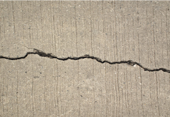
Flatwork cracks.
