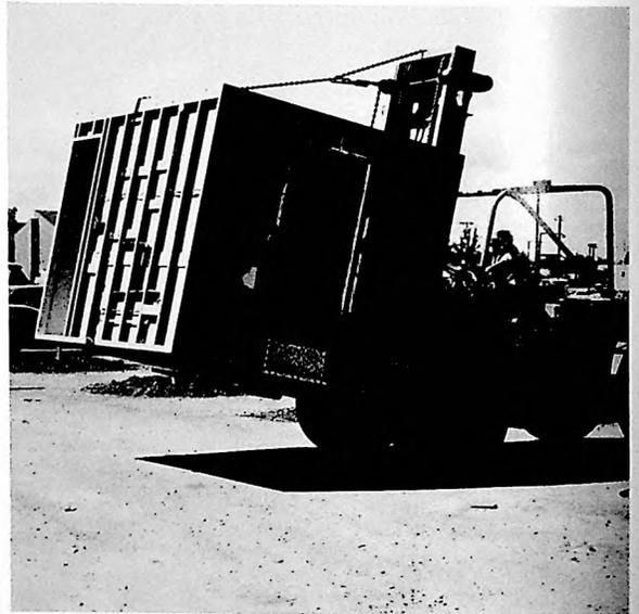
ALCOA'S MECHANICAL CORE MODULE BEING SHIFTED
