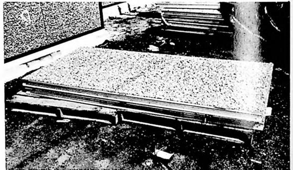
PANTEK'S PANELS STORED ON WOOD PALLETS. NOTE THE EXTERIOR SURFACE OF RIVERBED GRAVEL EMBEDDED IN EPOXY. VERY LITTLE TRANSPORTATION DAMAGE WAS ENCOUNTERED.
