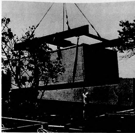
LIFTING FRAME WITH NYLON STRAPS
