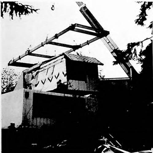
GUIDE ROPES ASSIST IN PLACING MODULES.
