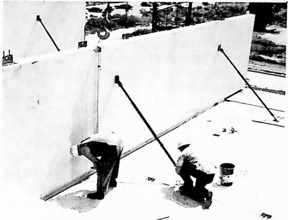
WALL-BRACING USED DURING ASSEMBLY OF DESCON'S UNITS
