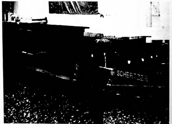
PNEUMATIC CUSHIONS ADDED TO PREVENT CRACKING OVER MODULE DOOR OPENINGS
