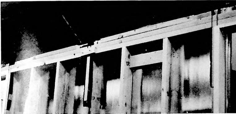
LIFTING STRAPS ATTACHED TO THE FIRST FLOOR WALL STUDS – NOTE SAW KERFS
