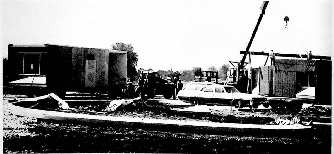
GENERAL ELECTRIC MODULE READY FOR PLACEMENT AT SITE. THE PICTURE WINDOW END WALLS WERE STRENGTHENED TO RESIST RACKING LOADS CAUSED BY RAIL TRANSPORT.
