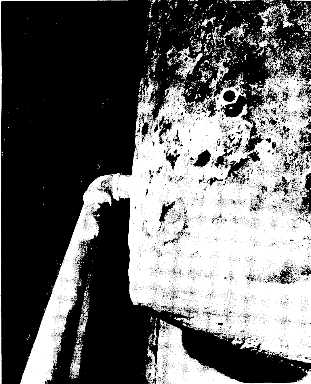
This view shows a few of the many holes in the metal of the tank top.
