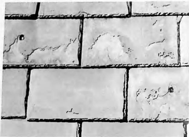
Figure 16 (Photo: Building Conservation Technology, Inc.)
