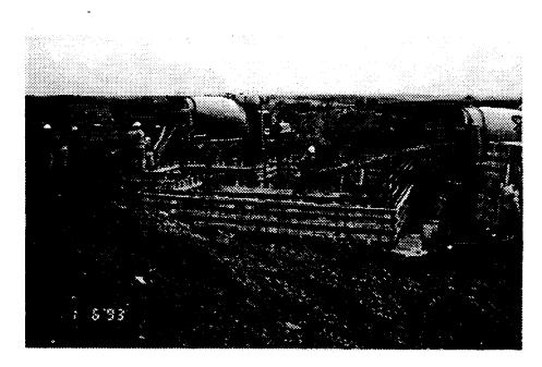
Figure 11. Foundation Walls Being Cast at the Eldersberg Site.
