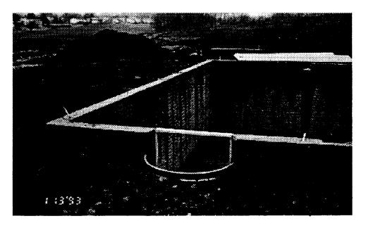
Figure 12. Completed Stemwall Foundation at the Eldersberg Site.
