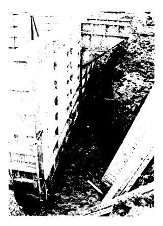
Figure 4. Eldersberg Demonstration House with Formwork Bearing Directly on the Ground.
